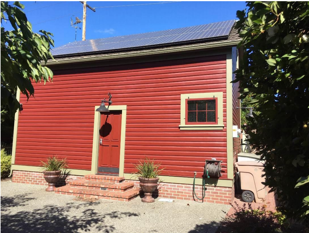
5 of 16. Front façade of carriage house.
