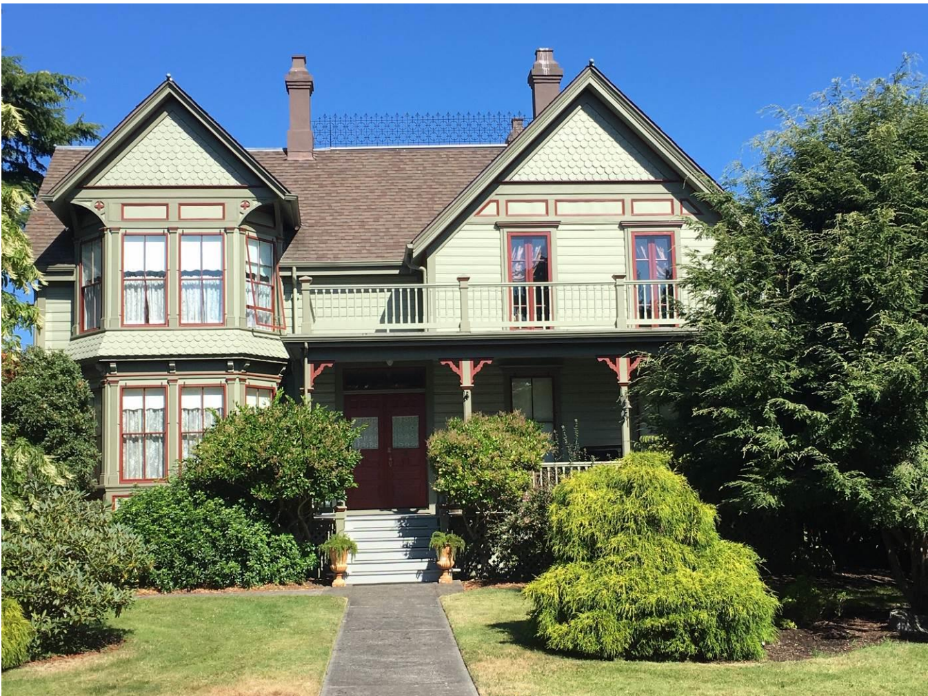
1 of 16 Front façade of house, southeast face of property, parallel to Franklin Street
