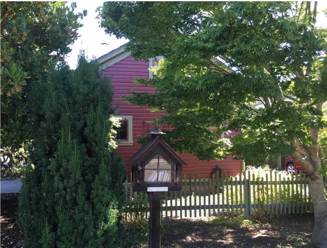
7 of 16. West side of carriage house.
