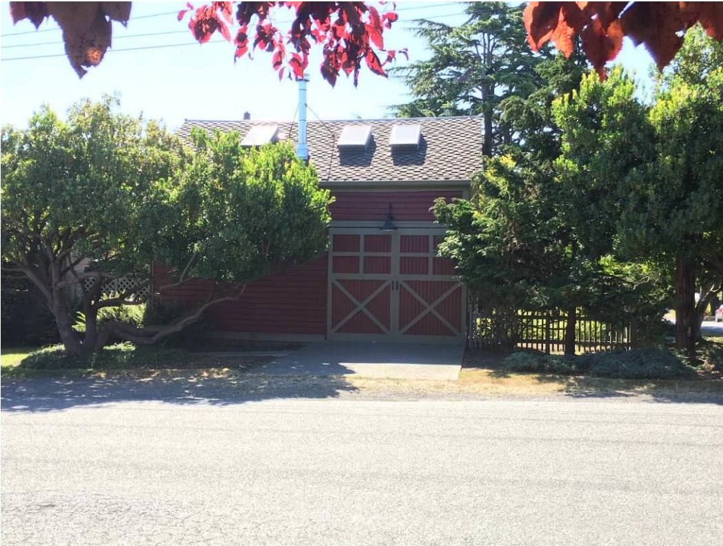
6 of 16. Rear of carriage house.
